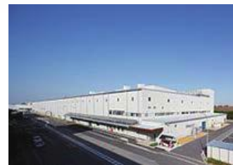
The waterborne paint Plant
